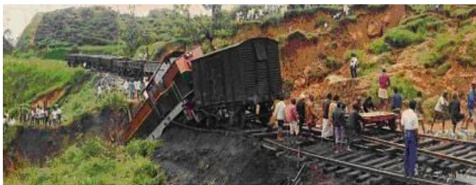
Picture: Earthslip at Watawala in 1992. Photo courtesy of National Buildings Research Organization, Colombo, Sri Lanka
