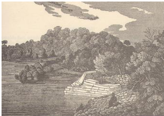
Graphic: Earthen bund and the Bisokotuwa or valve pit at the Kantalai Tank that was built in the 5th Century and later expanded in the 12th Century. The diagram has been reproduced from a wood-cut in John Davy's "Travels in Ceylon" produced in 1821.
